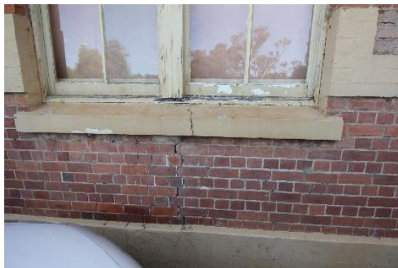
12: Window sills – showing deteriorated paint finish
