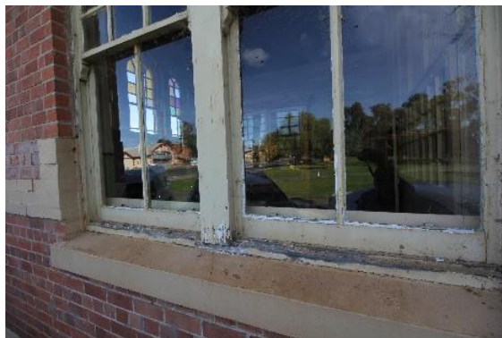
10: Window sills – showing deteriorated paint finish
