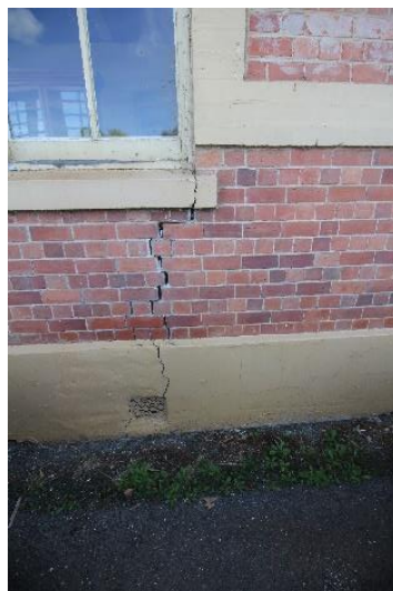
8: Cracking at brickwork – south façade
