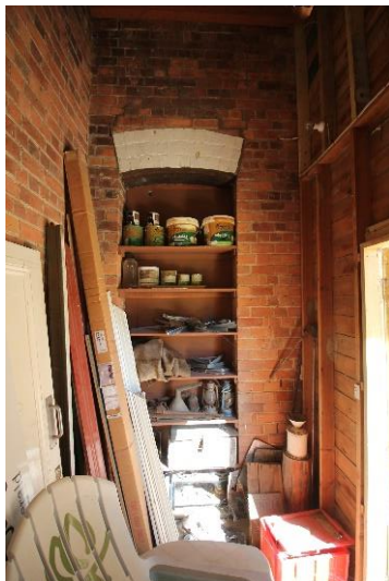
27: View to infill shelving at former door to become new egress
